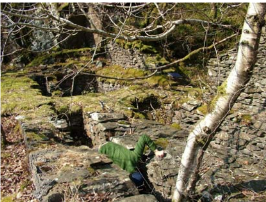
069) 40ft x 4ft wheel-pit – equipment compartments from south east corner
