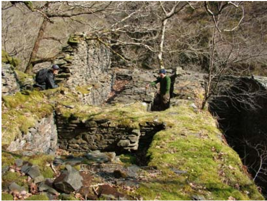
061) 40ft x 4ft wheel-pit – from tramway level
