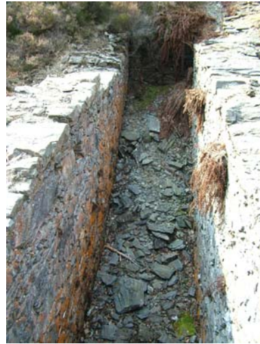
034) Dressing Floor – 30ft x 4ft wheel-pit (looking west)
