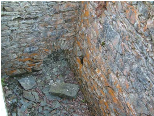
032) Dressing Floor – 30ft x 4ft wheel-pit (detail of drain arch)
