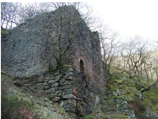
051) 40ft x 4ft wheel-pit – from river level
