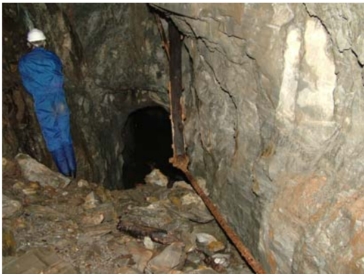
086) Deep Adit - shaft chamber looking west, pump-rod on right
