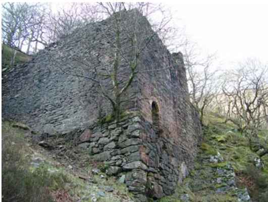
050) 40ft x 4ft wheel-pit – from river level
