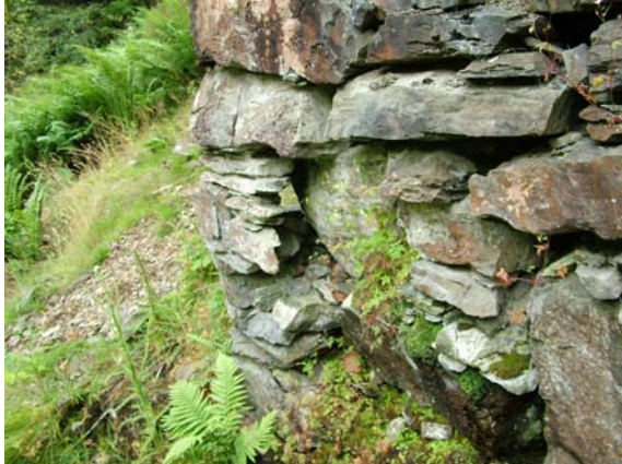
07) 40 foot wheel-pit - damaged stone south-eastern corner
