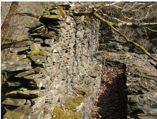
075) 40ft x 4ft wheel-pit – north east corner, compressor mounting base on right
