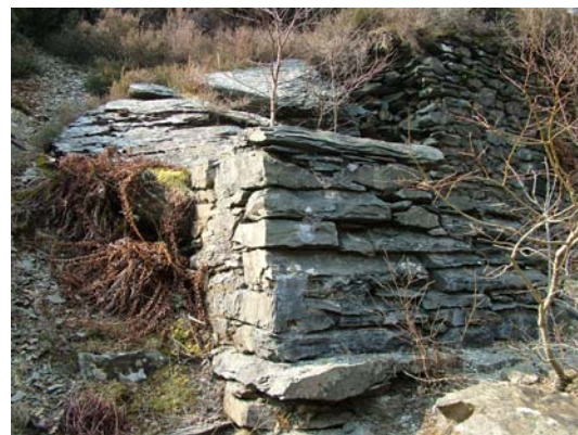
036) Dressing Floor – probable plinth for Blake's Stone Breaker (at west end of wheel-pit)
