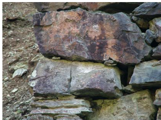
054) 40ft x 4ft wheel-pit – from river level (close up of damaged stone work)
