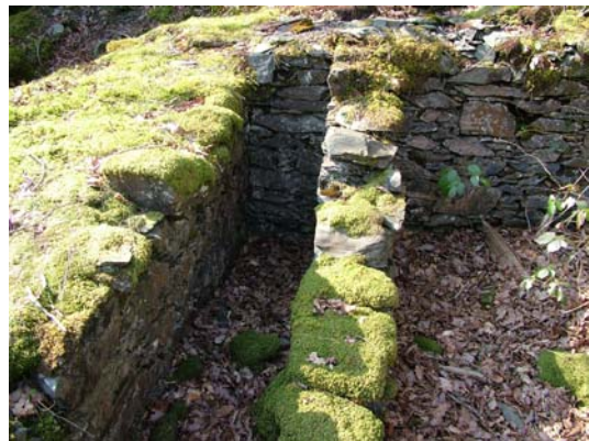
072) 40ft x 4ft wheel-pit – gearing pit on left, drum pit on right
