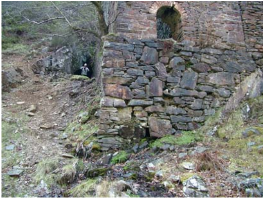
049) 40ft x 4ft wheel-pit – from river level, Deep Adit entrance on left
