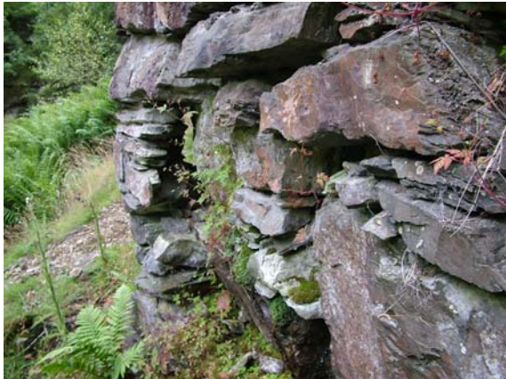
08) 40 foot wheel-pit - damaged stone south-eastern corner
