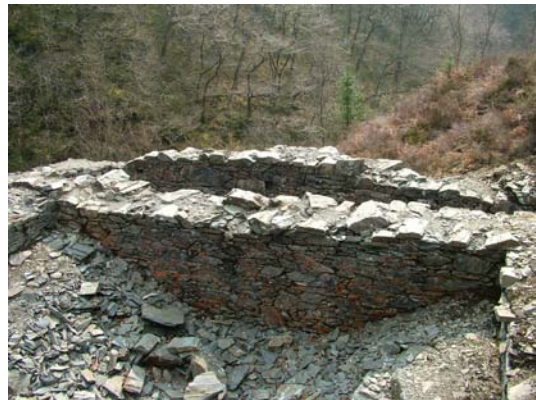
029) Dressing Floor – 30ft x 4ft wheel-pit (looking south)
