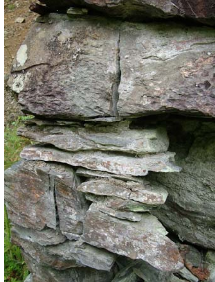
10) 40 foot wheel-pit - damaged stone south-eastern corner (close up)
