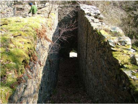
067) 40ft x 4ft wheel-pit – wheel compartment looking east
