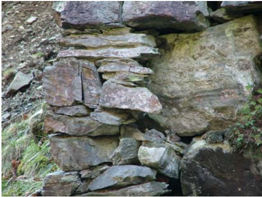
055) 40ft x 4ft wheel-pit – from river level (close up of damaged stone work)
