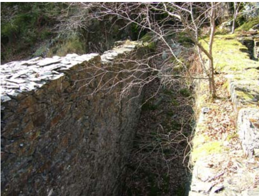
068) 40ft x 4ft wheel-pit – from tramway level (wheel compartment looking west)
