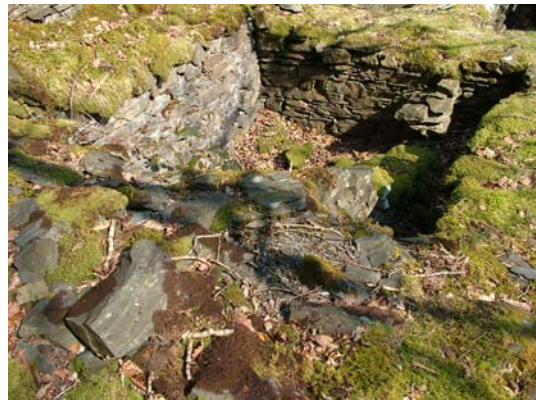
071) 40ft x 4ft wheel-pit – drum pit on left, gearing pit on right
