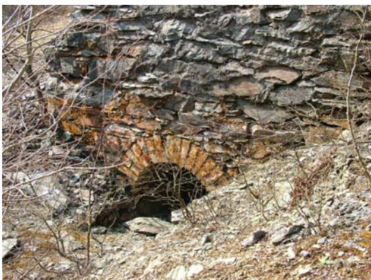
033) Dressing Floor – 30ft x 4ft wheel-pit (close up detail of drain arch)
