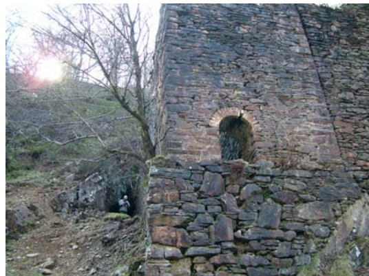
048) 40ft x 4ft wheel-pit – from river level, Deep Adit entrance on left
