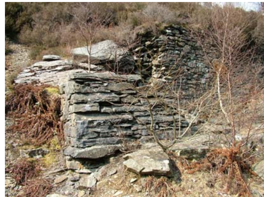
035) Dressing Floor – probable plinth for Blake's Stone Breaker (at west end of wheel-pit)
