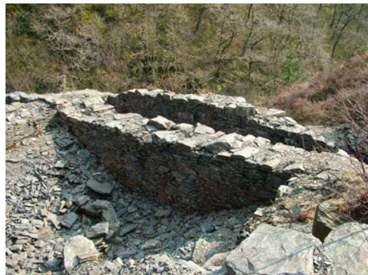
030) Dressing Floor – 30ft x 4ft wheel-pit (looking south)
