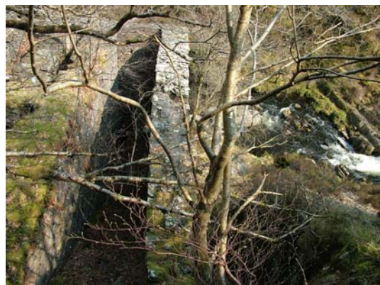
066) 40ft x 4ft wheel-pit – from tramway level
