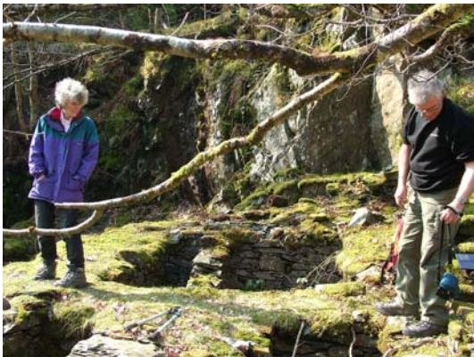
074) 40ft x 4ft wheel-pit gearing pit on left, drum pit on right
