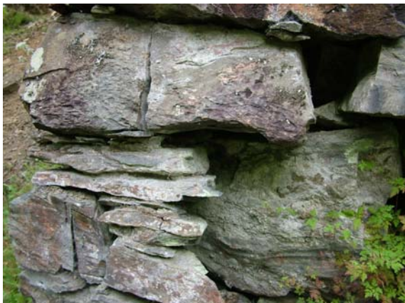
09) 40 foot wheel-pit - damaged stone south-eastern corner (close up)
