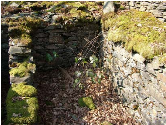
073) 40ft x 4ft wheel-pit drum pit
