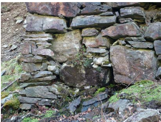
057) 40ft x 4ft wheel-pit – from river level (close up of damaged stone work)
