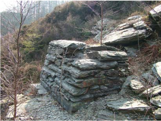
037) Dressing Floor – probable plinth for Blake's Stone Breaker (at west end of wheel-pit)
