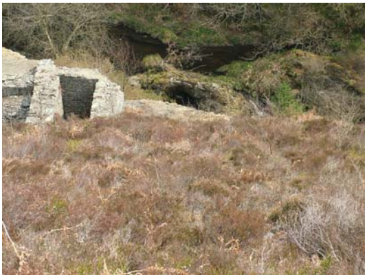
008) 30ft x 4ft wheel-pit and base of incline (on the right hand side)
